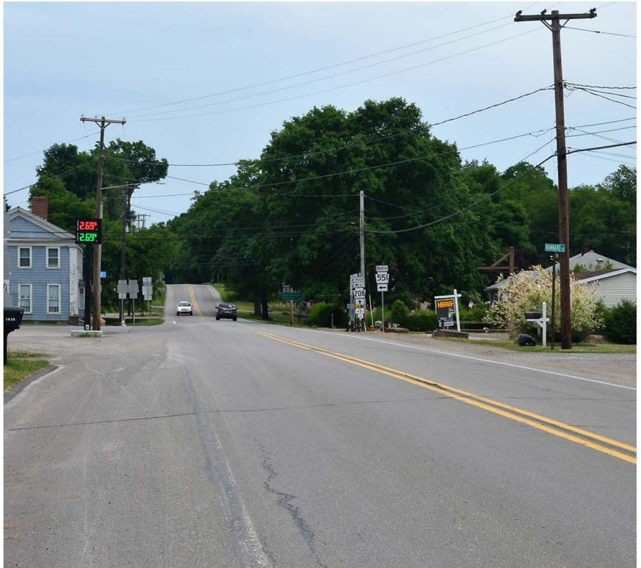
A complete street in a rural community can be as simple as providing wide shoulders to allow for safe bicycling, walking and Amish buggies.
