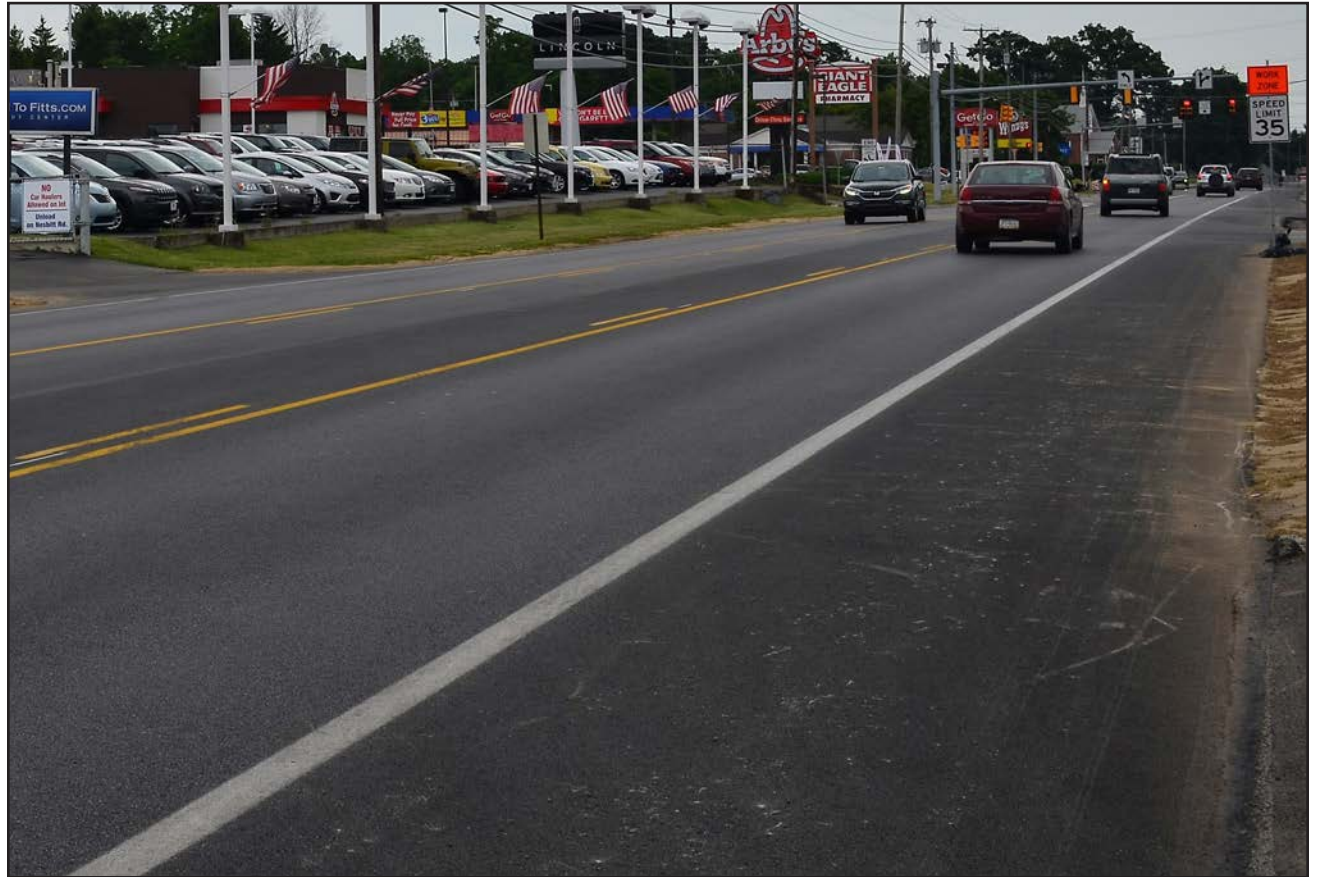
Example of 8' shoulders along SR 18 in Neshannock Township. Representatives of Amish and cycling communities cited this as a preferred design for corridor improvements.
