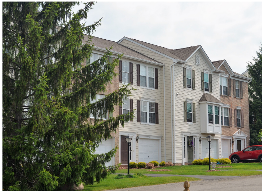
New townshouses in Shenango Township
