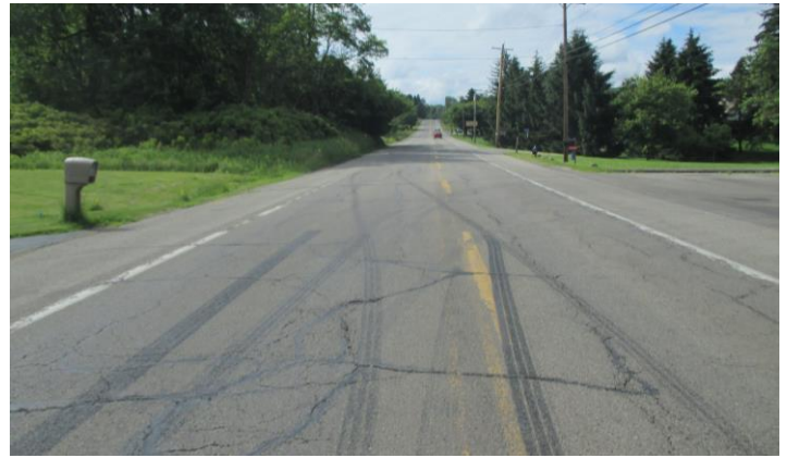
SR 65 Double Yellow Pavement Markings Worn, Revealing Old Passing Zone Pavement Markings Underneath
